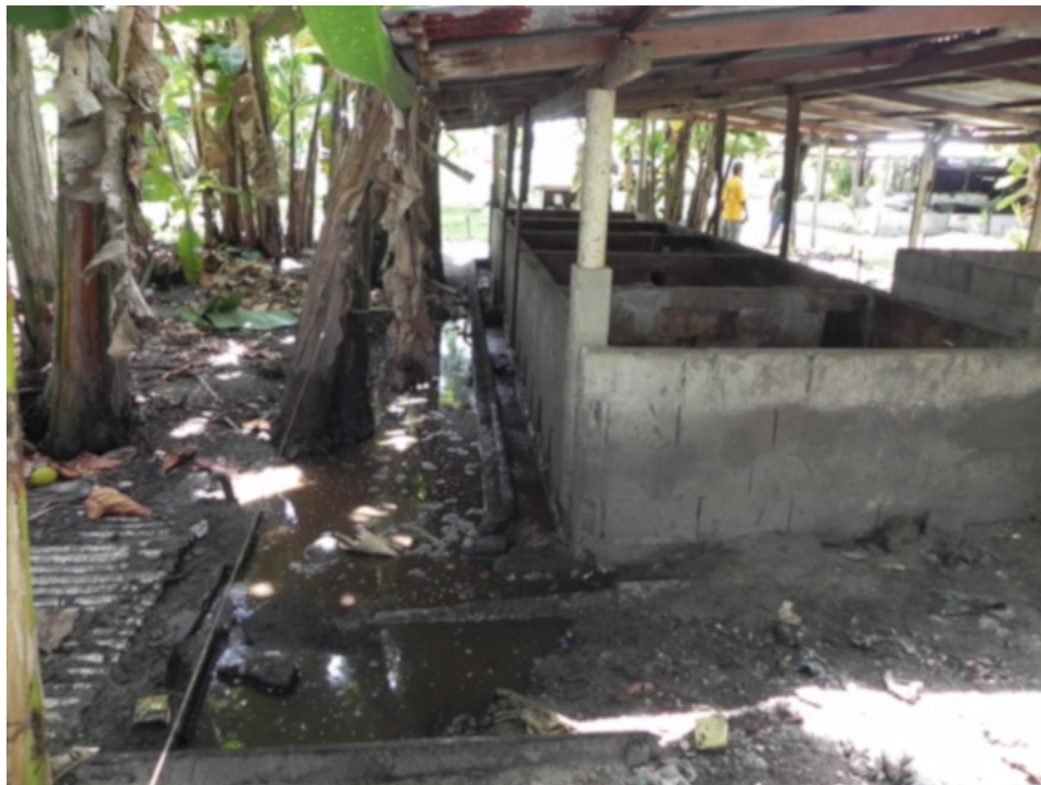
Figure 2. Piggery effluent backup at the inlet to a cesspool.
