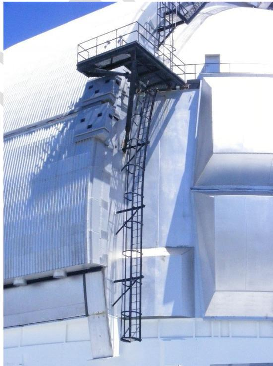
Figure 2. Photo of one of the four Enclosure ladders longer than 24 feet that require lifelines.
