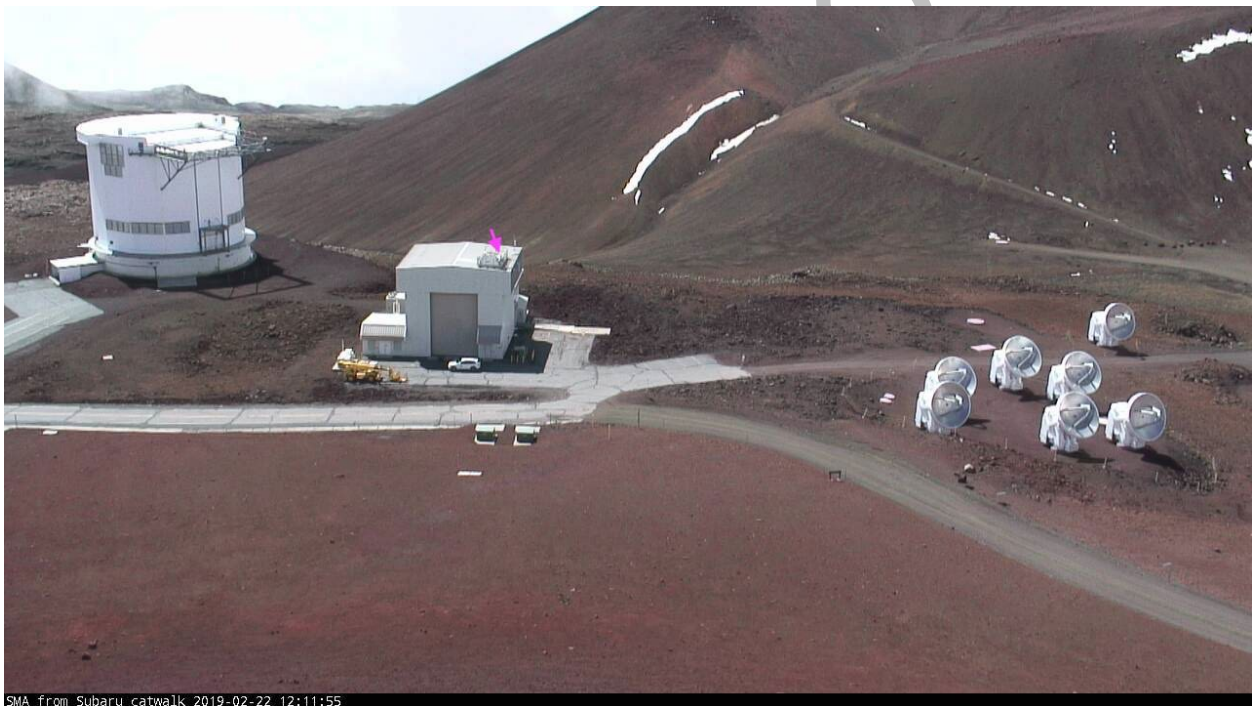
Figure 1. The SMA hangar (center), JCMT (left), and SMA antennas (right) viewed from the Subaru catwalk. The existing AMOS is located in the center of the platform on the roof of the SMA hangar. The meteorological instruments will be installed near the north corner of the platform (arrow).
