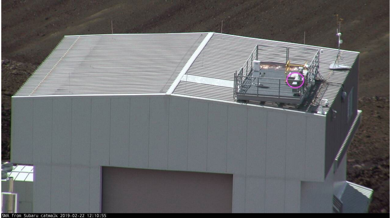
Figure 2. Magnified view of the SMA hangar roof from the Subaru catwalk. The existing AMOS is located near the center of the roof platform. The meteorological instruments will be installed near the north corner of the platform (circle). The existing mast outside of the platform will be removed.
