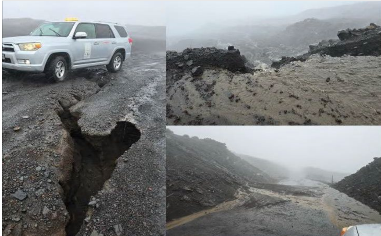
Figure 13. Hurricane Hone Damage.
