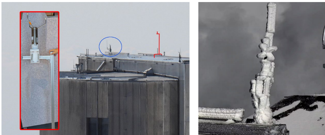
Figure 10: [Left] current (blue circle) and proposed location (shown in red lines, see also Figure 11) of the existing anemometer at the top of the Subaru Telescope enclosure. The inset picture is the new ultrasonic anemometer. [Right] Current anemometer sometimes freezes up by harsh environment of the summit area, like the picture here. The new anemometer does not have any movable parts with heater, so we expect it is much more tough even under such condition.
