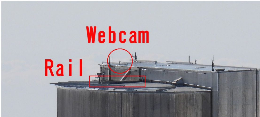
Figure 9: the position of the webcam which we propose to put the IR illuminator. This is a zoom-in view of the Subaru Telescope Enclosure.
